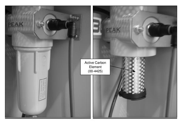
The filter housing is removed by un-screwing in a counter clockwise direction.
